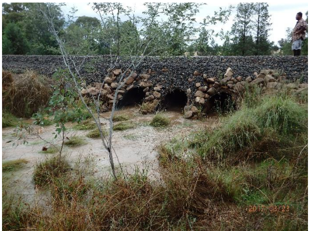
Plate C1.18 – Downstream side of the three 1050 mm diameter corrugated pipes beneath the railway to the east of Haynes Street (Photo taken at 09:12 hours)
